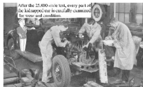
After the 25,000-mile test, every part of the kidnapped car is carefully examined for wear and condition.
